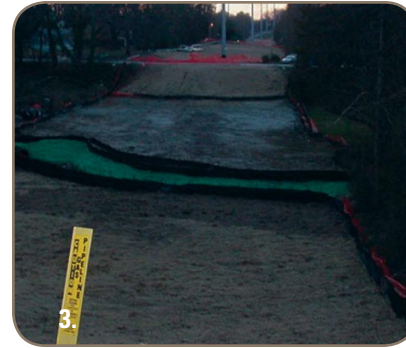
3. Photo 3 shows how the pipeline trench will look shortly after it is re-covered. And Photo 4 shows the area after relandscaping.
