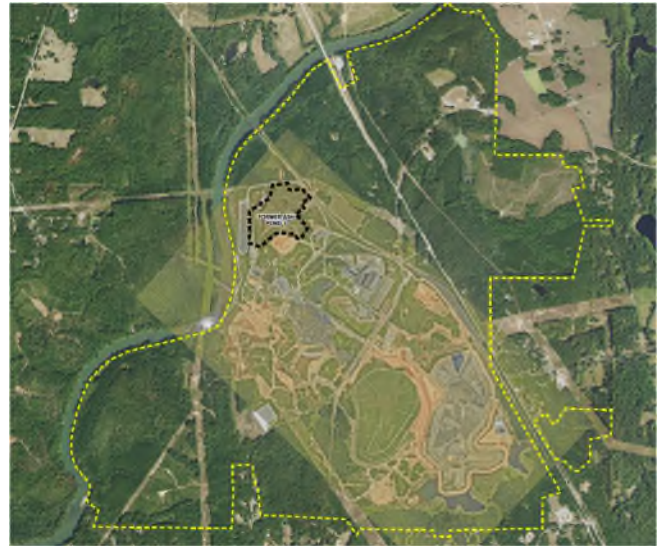
Plant Yates and the site
