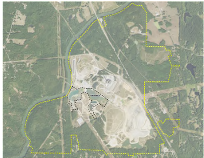
Plant Yates and the Site
