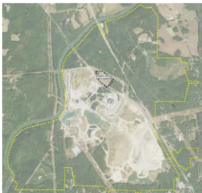
Figure 1. Plant Yates and the Site
