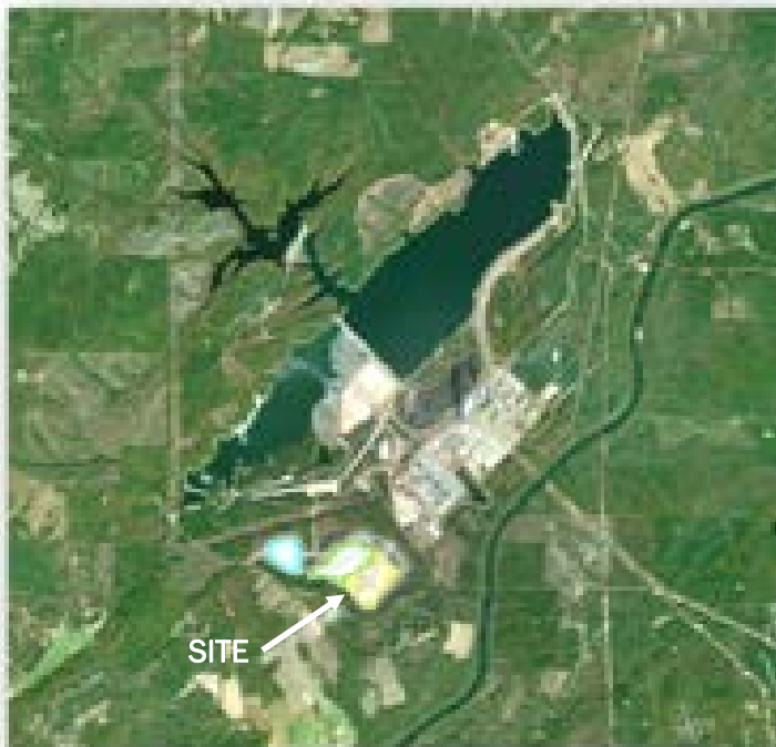
Plant Wansley and Plant Wansley Landfill
