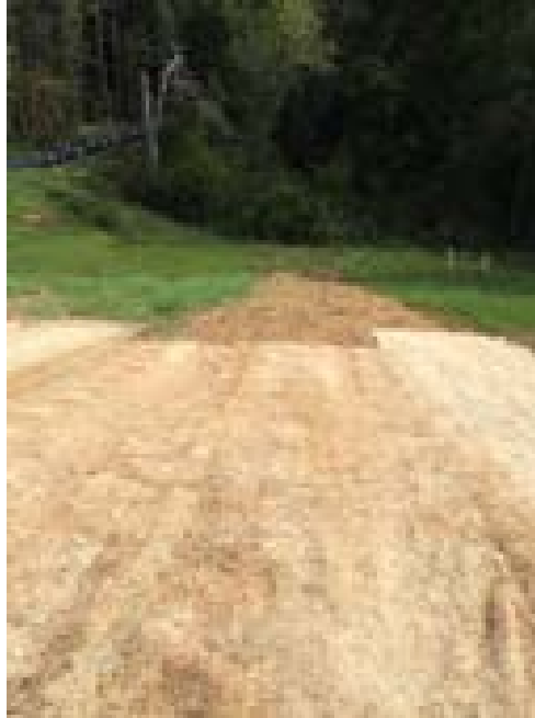
Exhibit 3 Embankment Repair Uphill from GWC-14.
