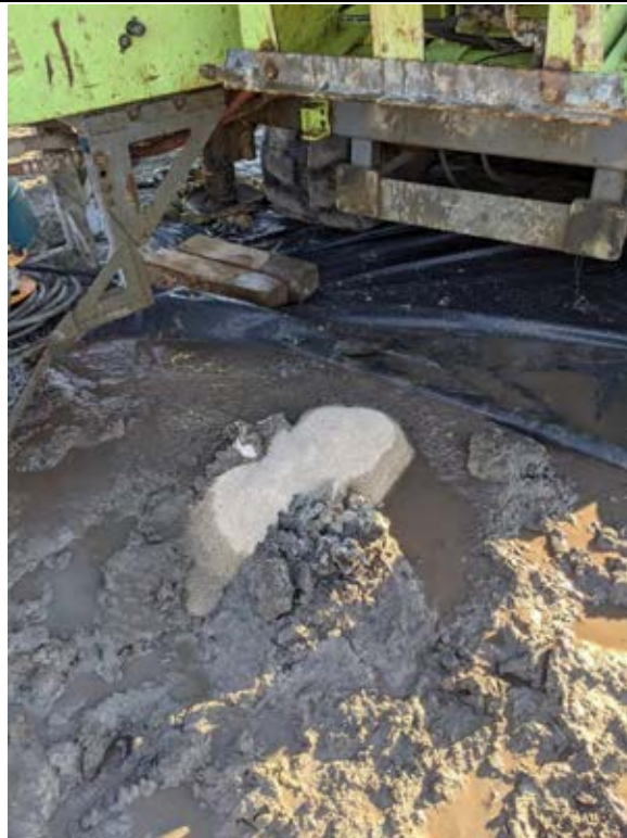
Finished backfilling 25 ft, 9-inch borehole from bottom of ash pond to ground surface.
