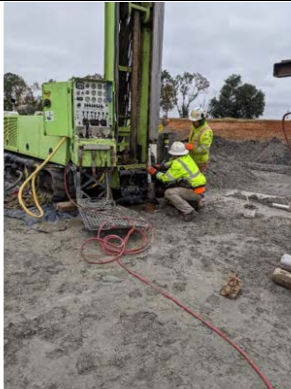
Removing augers and well casing after backfilling with grout.
