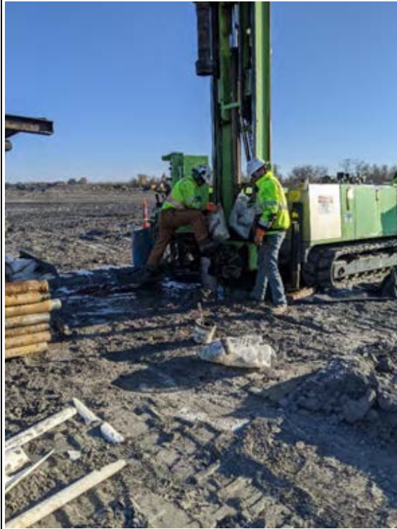
Backfilling 25 ft., 9-inch borehole through ash with sand.
