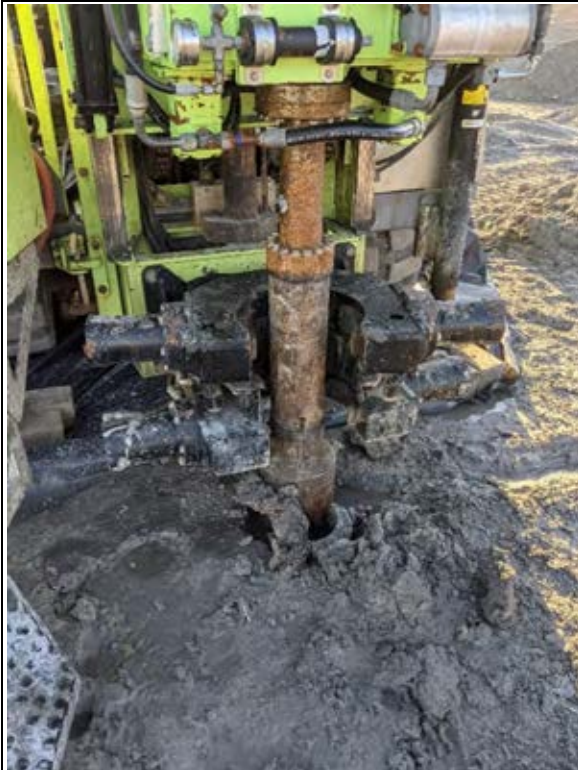
Drilled down to 25 ft. to bottom of ash pond.
