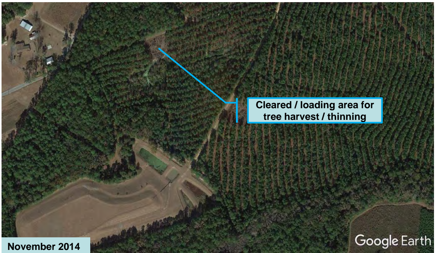
Figure 2. Aerial Imagery Comparisons 2012 / 2014 Plant McIntosh Monofil No. 3 Rincon, Effingham County, Georgia
