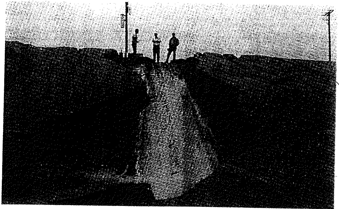
FIGURE 13.15 Sand Layer Failure along Sideslope Caused by Seepage Force
