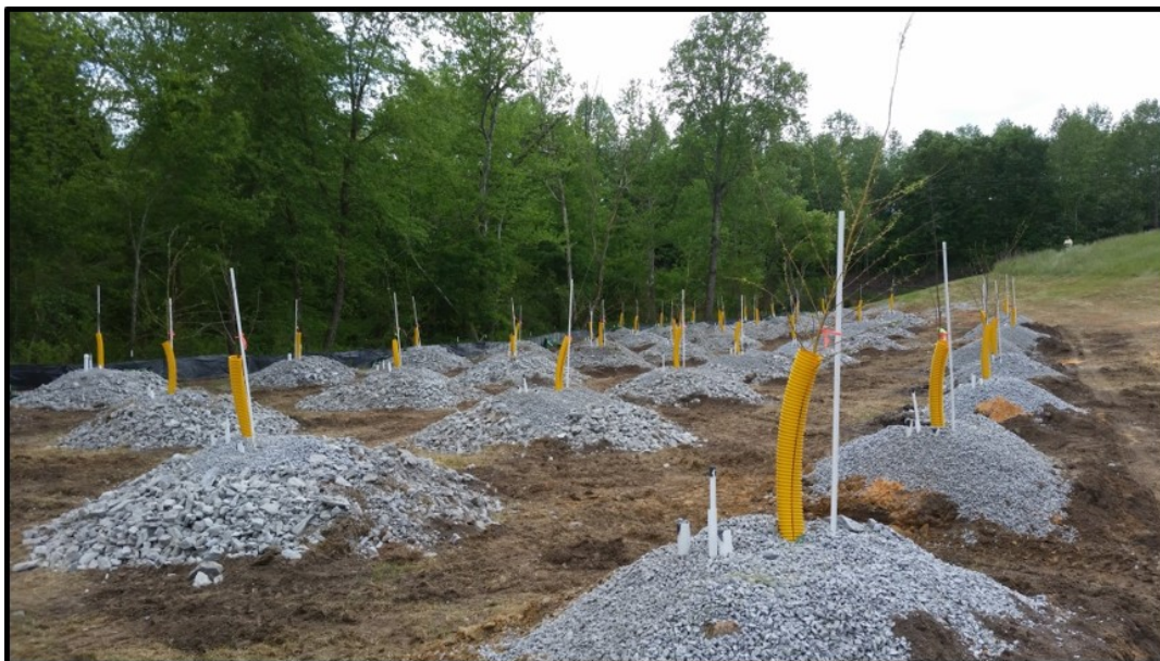
Figure 2: Newly completed TreeWell units at North Carolina site.
