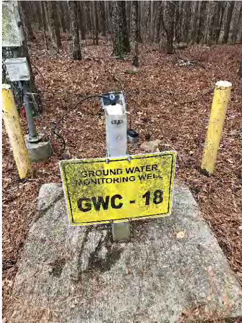
Photo #2: Overall condition of well
