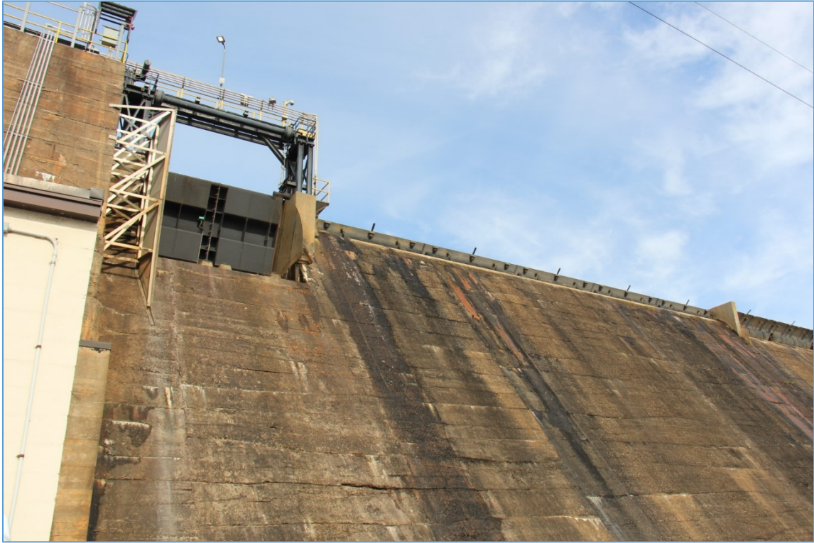
Figure 13. View of spillway face and spillway trash gate, looking northeast, December 2, 2019.
