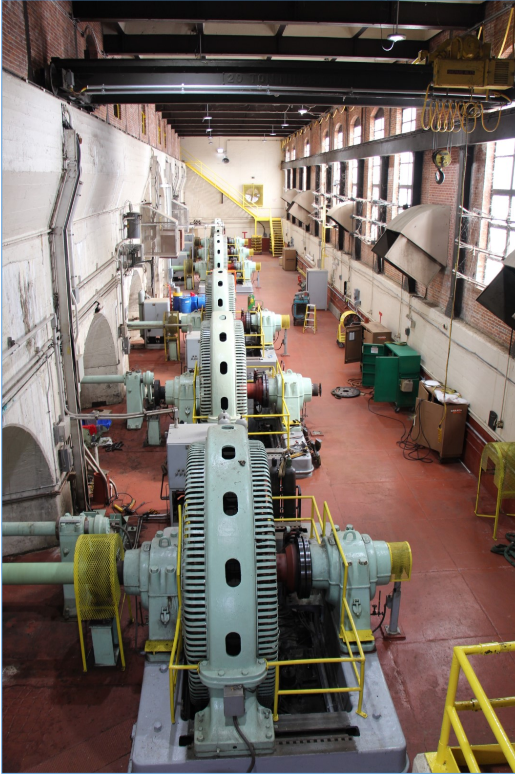
Figure 15. View of powerhouse main generating floor, looking southeast, December 2, 2019.
