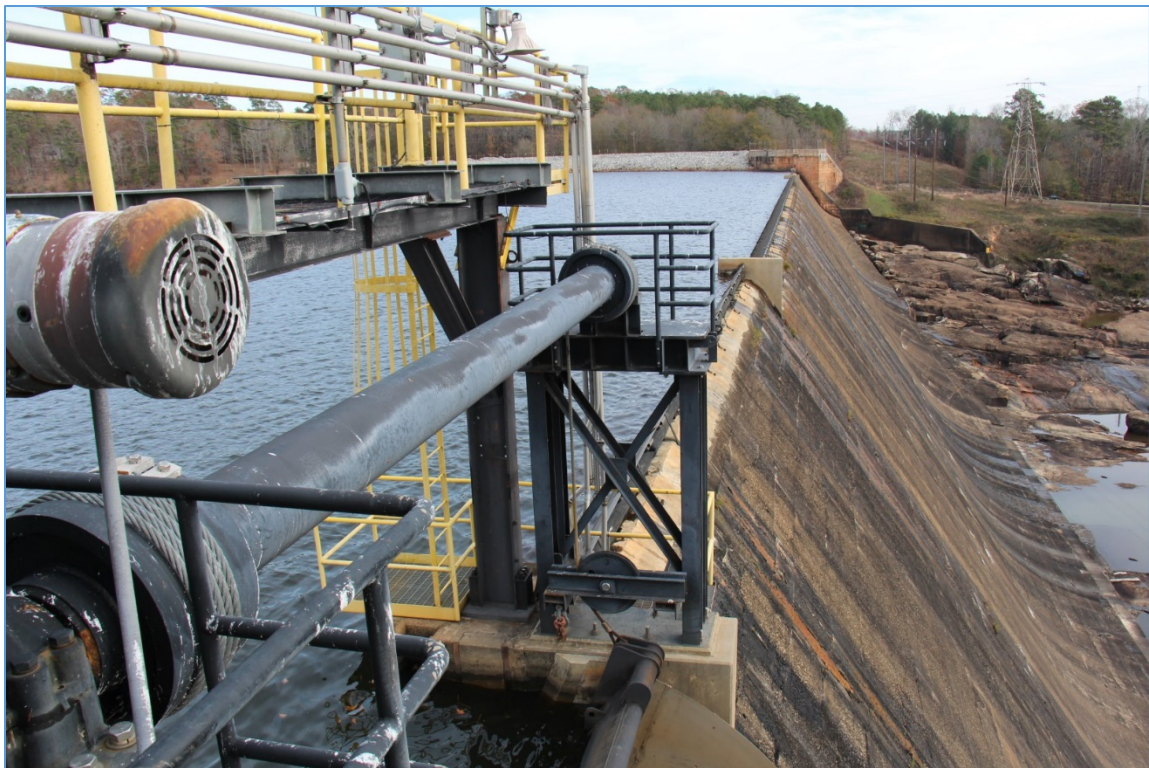
Figure 14. Crest of dam and spillway, December 2, 2019.
