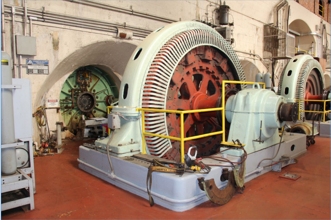
Figure 16. Generating Unit 1, looking northeast, December 2, 2019.
