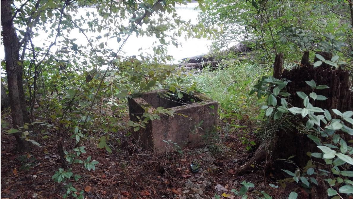
Figure 17. Possible remnant of the Bug House noted within 9BS18, facing north.
