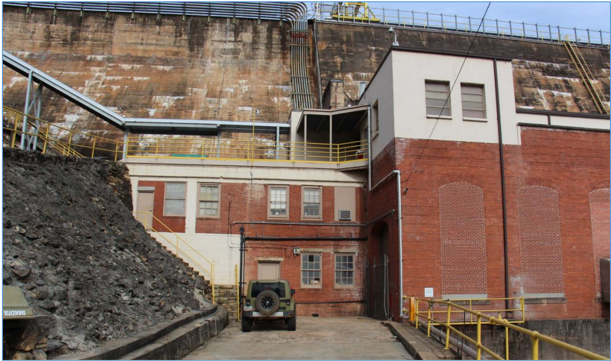
Figure 11. Administration area at west end of powerhouse, looking northeast, December 2, 2019.
