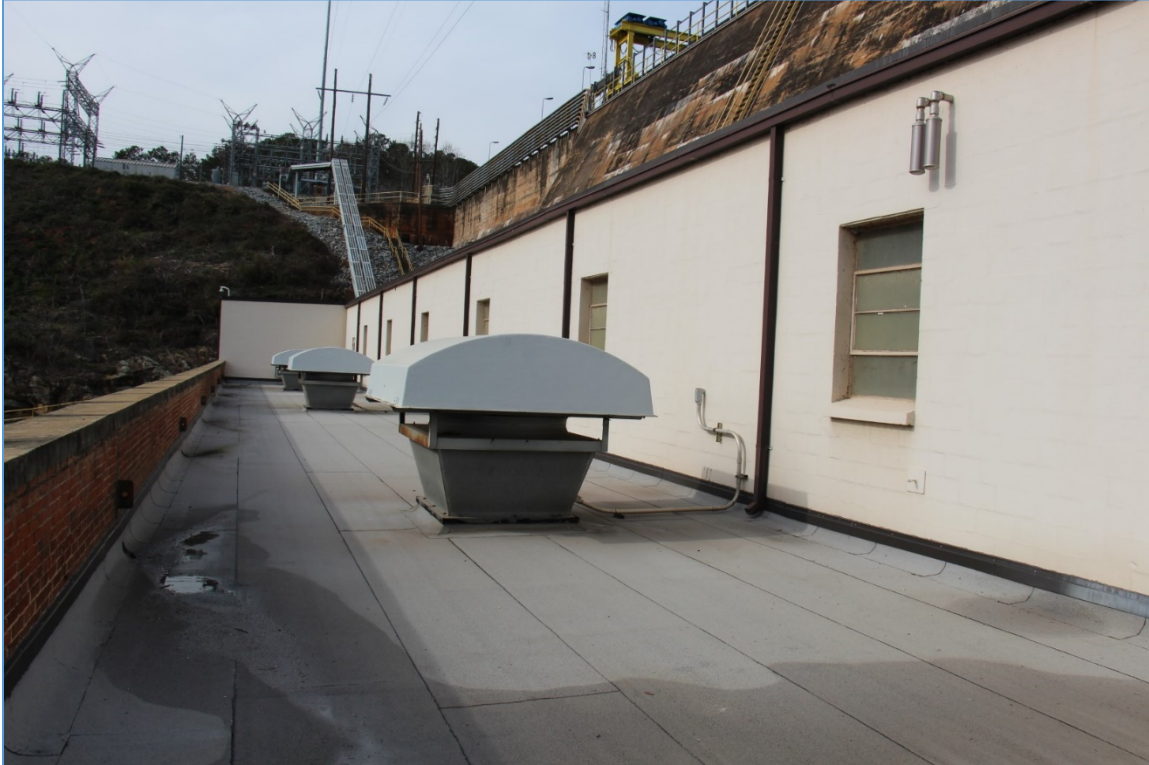
Figure 18. Exterior view of second floor, looking northwest, December 2, 2019.
