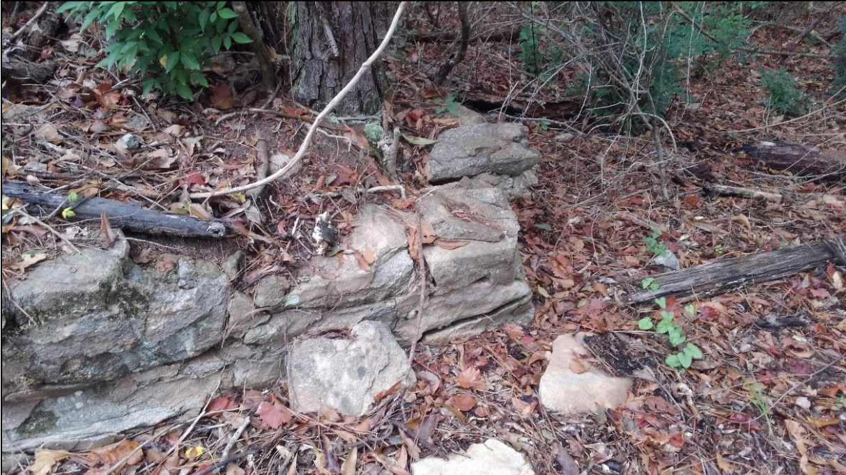
Figure 18. Northwest terrace wall corner at sit 9BS18.
