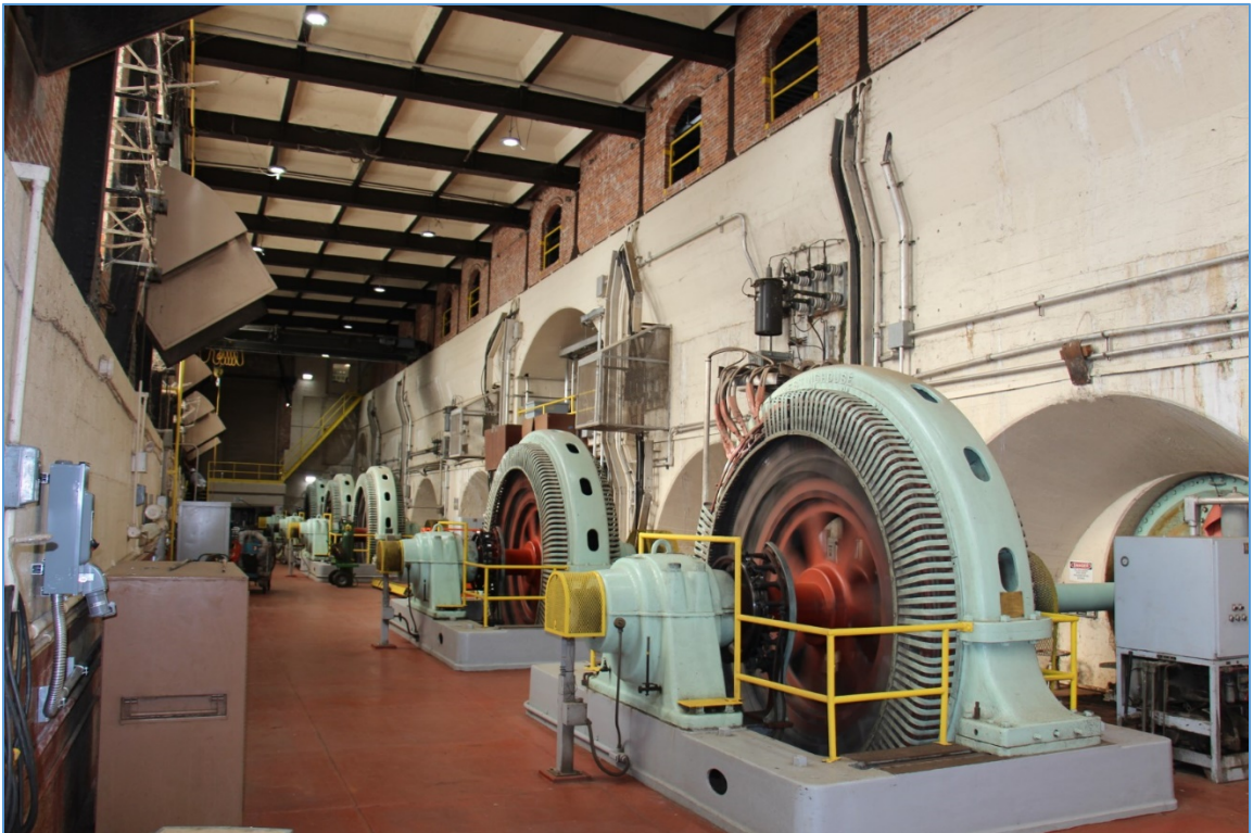
Figure 17. View of main floor, looking northwest, December 2, 2019.
