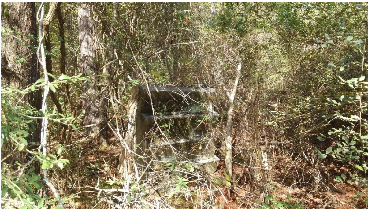
Figure 10. Concrete stairs at Site 9BS17.
