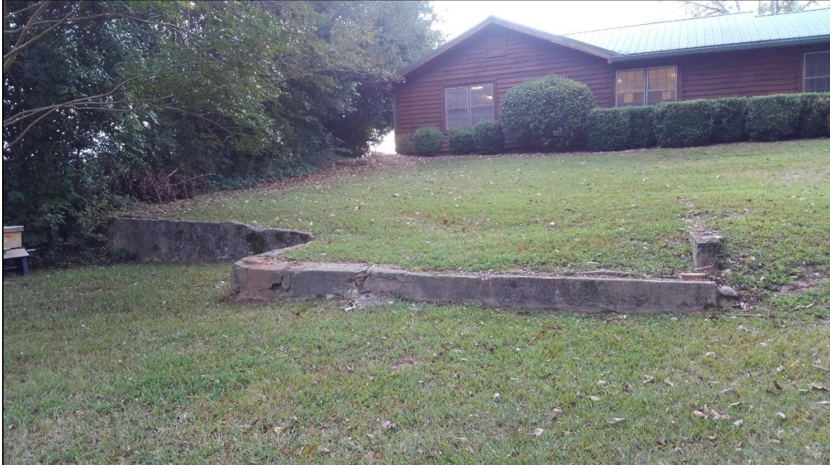
Figure 21. 9BS20 in 2019, facing east.
