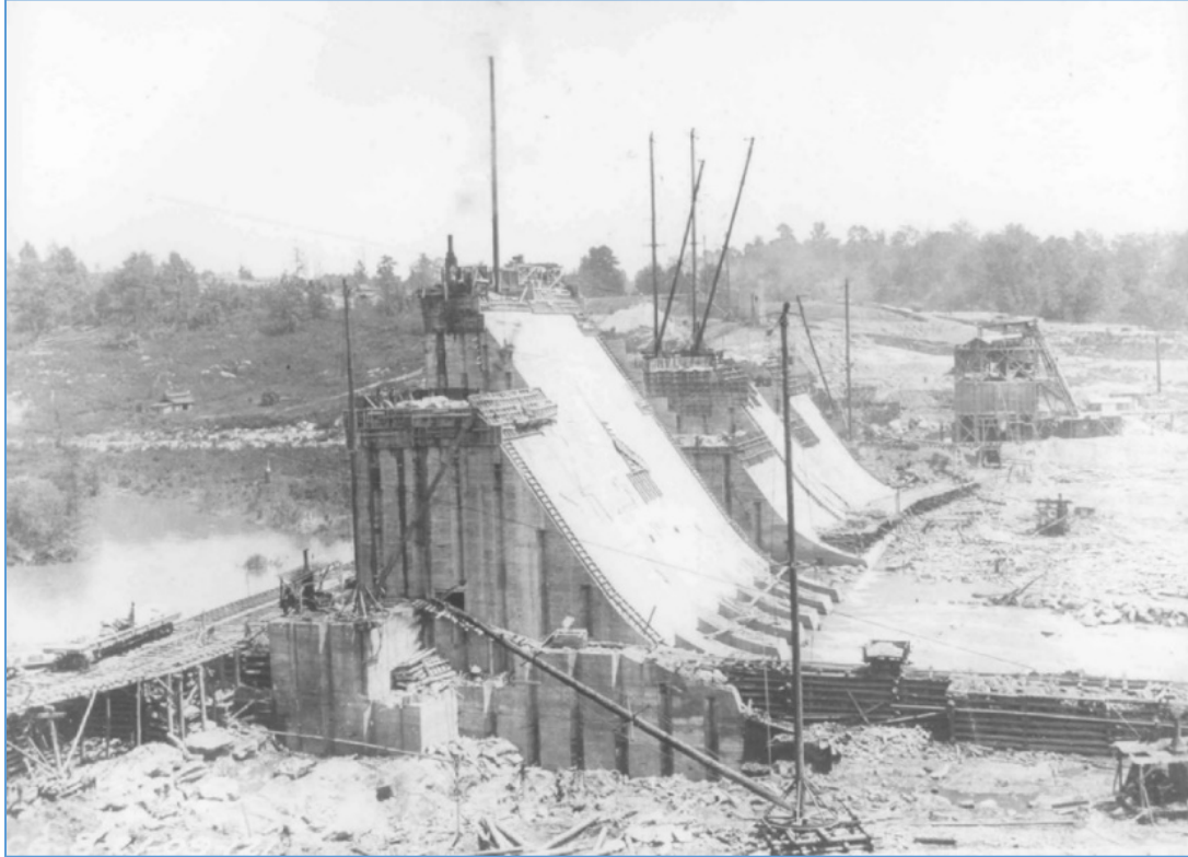
Figure 2. Lloyd Shoals dam construction, looking east, August 1909 (Courtesy of Georgia Power).
