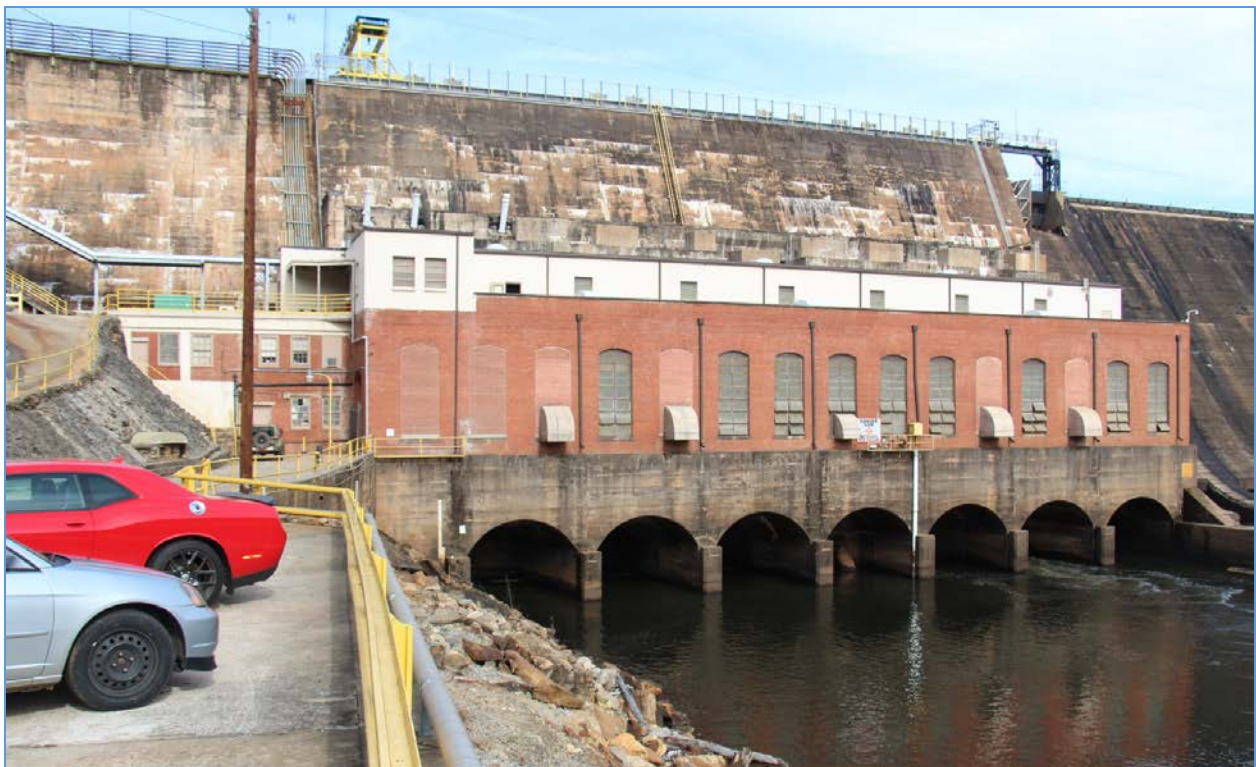
Figure 10. View of the powerhouse and non-overflow section of dam, looking northeast, December 2, 2019.
